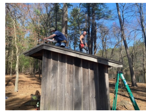
Adult volunteers Ed Hoffman and Mike Nipoti installing the new shingles.
