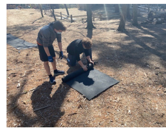
Fellow scouts Jacob Nipoti and Brady Burton cutting the new shingles for the roof.
